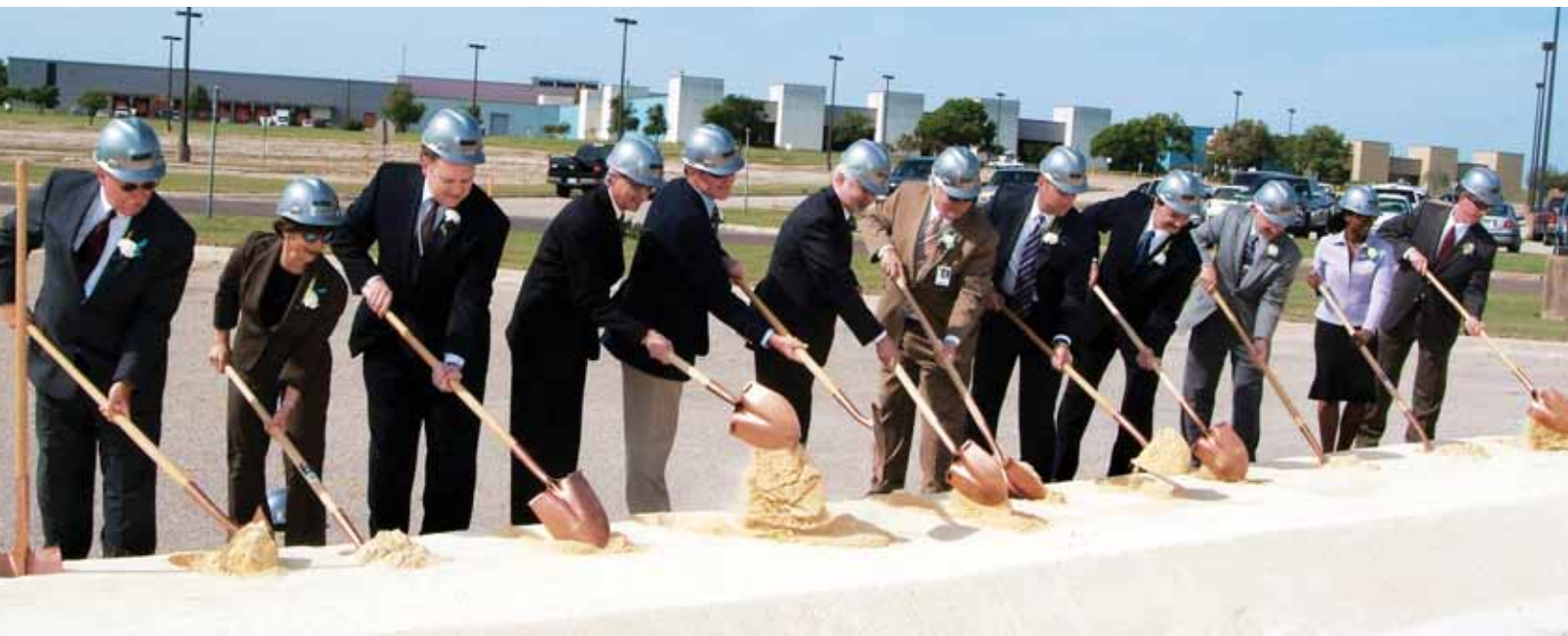
Scott & White leaders break ground at the site of a new long-term acute care hospital.
